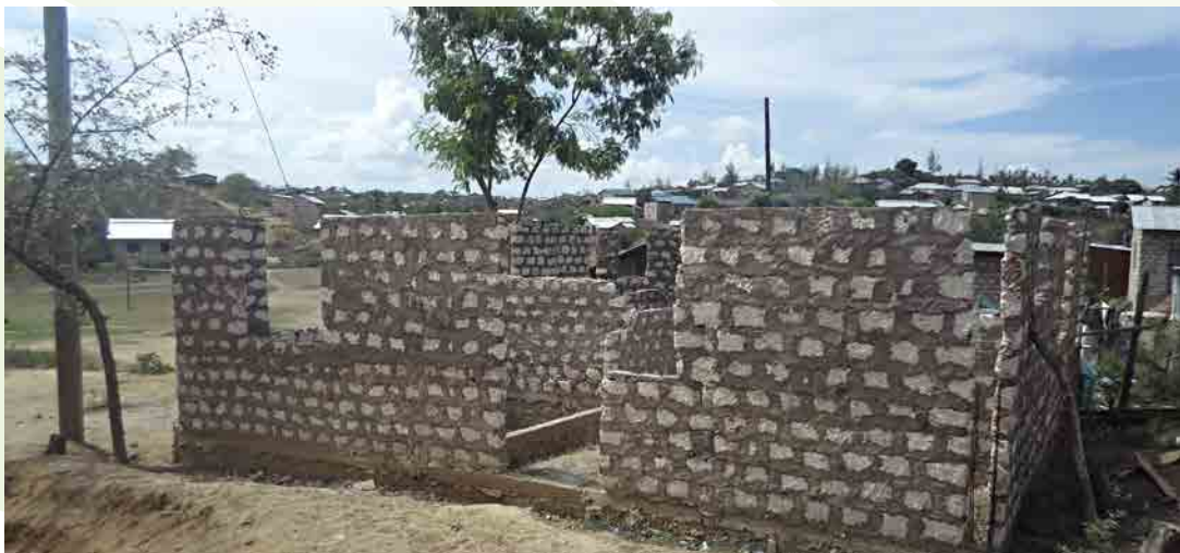
An abandoned structure in Kadongo Mwembeni area
